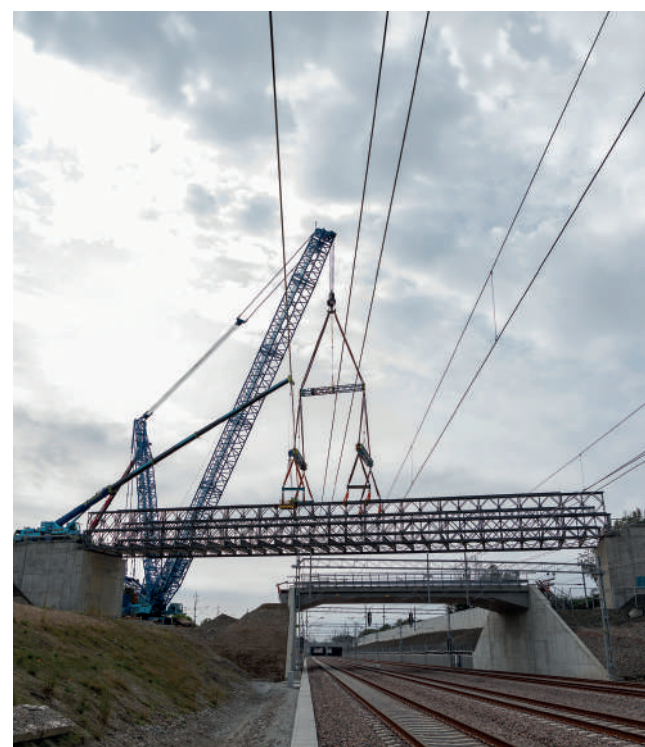
Removal of the 150-tonne Åkarp bridge in Sweden. Picture: Niclas Franzén, OHLA/NCC.
